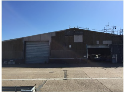
OUTSIDE BUILDING TO DATE 14/06/2017
